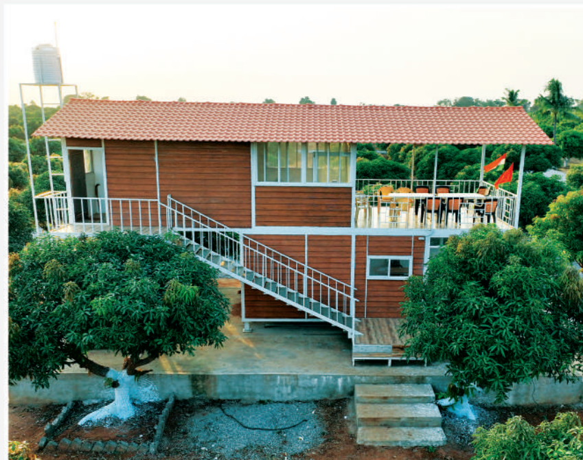
Duplex Wooden House
