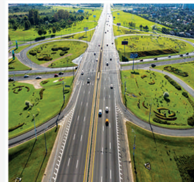
Adjacent to 6 lane NH-44 Hyderabad to Bangalore Express Highway
